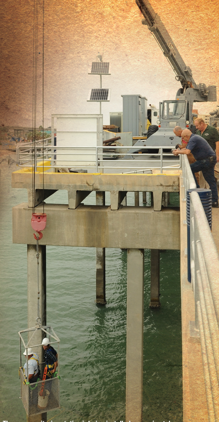
The new monitoring station is being installed approximately 25 feet above sea level to protect equipment from high-water events such as storm surges, which have historically damaged or destroyed data collection systems.
