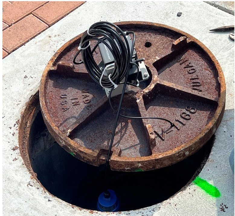
An AI-powered monitoring device, installed on a sewer line on the TAMU-CC campus, collects data that could lead to smarter, more efficient infrastructure maintenance.
