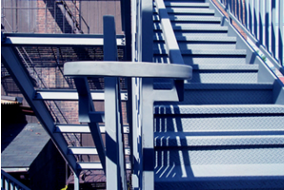
Round contour handrail provided on multi level units
