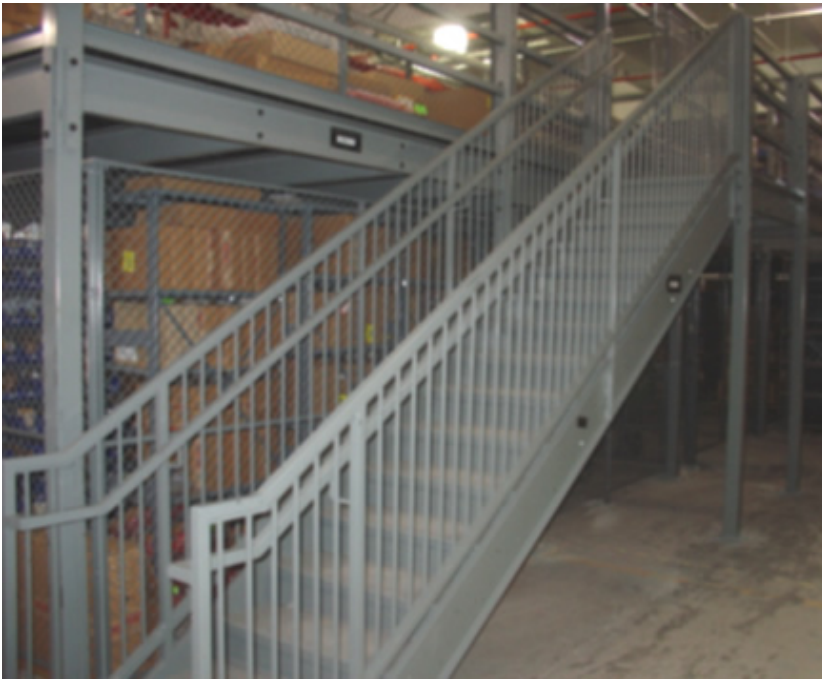
IBC stair with vertical balusters provides complete code compliance.
